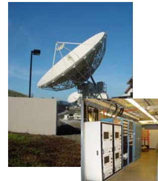
4 Signal Generator System/ Ground Earth Stations
